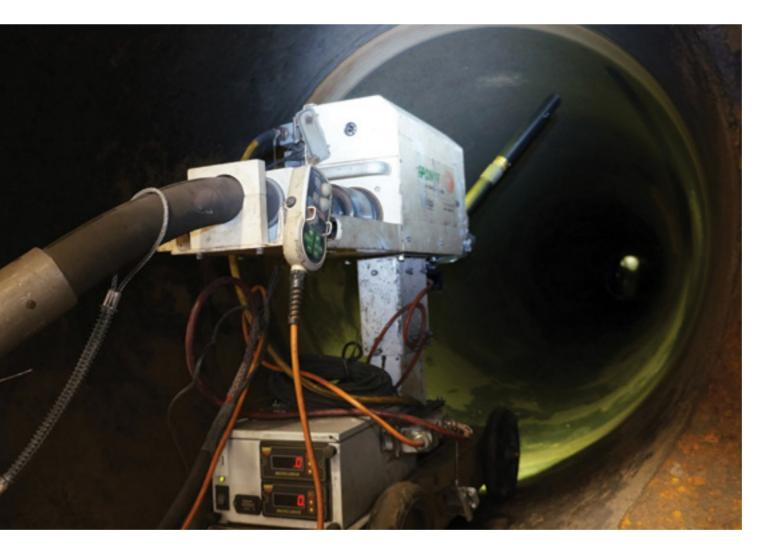
FIG. 4: Robotic abrasive blasting was a safer option for the crew, allowing for reduced man hours spent in the confined space of the pipe.
