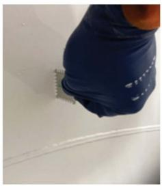
FIG. 7: The crew performed QC testing that included visual inspection, wet film thickness testing, dry film thickness measurements and holiday testing in accordance with NACE SP0188.
