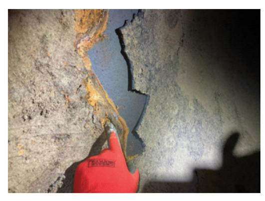
FIG. 2: The crew had their work cut out for them as the coal-tar enamel had failed in areas, leaving behind corrosion in the 60-inch raw water pipe.
