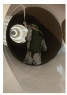
FIG. 6: Using spray application equipment, the crew applied three coats of an 80%-solids epoxy coating specially designed for application in pipes and tanks containing potable water, wastewater and salt water, in contrasting colors (white, blue and white) at dry film thickness of 7 mils per layer. In between the first white coat and the blue coat, the crew applied a stripe coat to all edges, welds and transition areas.
