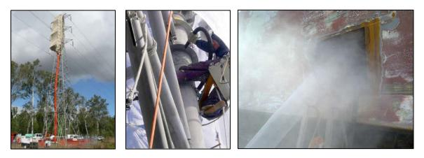
Figure 21 - Left: Environmentally sensitive project utilizing composite abrasives Middle: Note low dust blasting with Composite abrasives Right: Representative example of fugitive emission with mineral abrasive (garnet)
