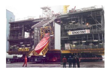
Coating engineers with a Netherlands manufacturer of offshore platforms searched for a method to repair weld seams. Welding, during assembly of the rig causes staining and damage to prepainted parts. Engineers wanted a repair process that would cause less damage to sensitive surrounding parts of the rig and equipment already in place. They chose Silver Sponge Media™ abrasives because of the following process characteristics:
