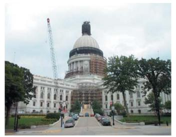
Wisconsin state architects required a cleaning method that could remove exfoliation from decaying granite surfaces of the Wisconsin State Capitol (WSC). The project called for cleaning stone ornaments and statues, balustrades, columns, walls, stair-treads, and one of the world's three granite domes.
