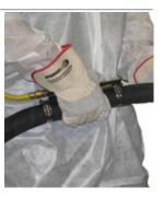
IF no air is felt exiting red air line, trace air flow operation through Twinline and Deadman Handle checking for obstructions or leaks.
