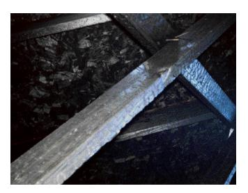
Immediately following a plant fire, facility owners turned to Moore Restoration to remove soot and charred residual coatings. The facility had to reopen as soon as possible. The char and contamination layers to be removed from the pine wood trusses and plywood sheets covering the ceiling were from 5 to 75 mils thick. Moore Restoration's decision to use Silver Sponge Media™ #80-grit abrasive and the Sponge-Jet Sponge Blasting™ System to restore the surface was based on a few key challenges:
