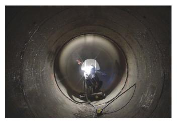
ABOVE A Robotic carts tend to be scene stealers, but the heavy lifting on this project was accomplished by a crew from Structural who hand-rolled and troweled a proprietary, multi-layered, reinforced V-Wrap 700 epoxy coating system.
