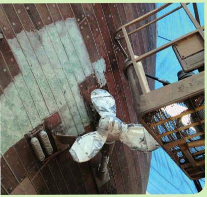
The conventional blast media bonded to sponges did the trick; removing the old bottom paint without compromising the caulking or over-profiling the hardwood
