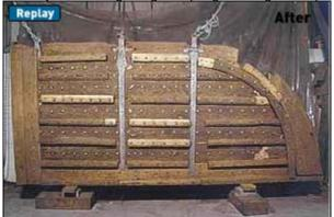
restoration as part of celebrations of 700 years of worship there. The gates themselves date from the 14th Century and are of oak, which has been heavily coated with bitumen and lime. Both wear and attack by wood boring beetle had inflicted considerable damage on the material.
