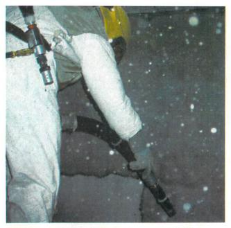
The tank's 2,500 square foot surface area had to be blasted in roughly 8' x 10' sections to prevent the exposed steel from flash rust. Blasting Silver 30 Sponge Media with aluminum oxide through SpongeJet's 85-L Feed Unit and 35-P Pneumatic Recycler, the crew brought the steel surface to the specified SSPC #6/NACE 3 standard for commercial blast surface preparation. Then they immediately primed the freshly blasted sections with Tnemec's two-component Tneme-Zinc 90-97 zinc-rich primer.
