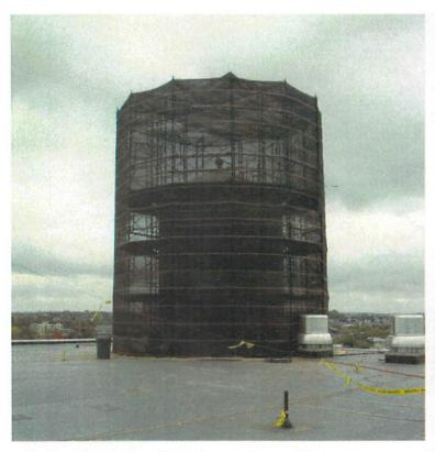
Prior to E.M.C.'s arrival on the job, scaffolding had been erected on the rooftop surrounding the tower. Wooden trusses were placed on top of the scaffolding. To enclose the tower and prevent overspray, finely woven mesh tarps were draped over the trusses and around the tower's perimeter. With the scaffolding and tarps in place, all of the necessary materials — including the sandblasting equipment — were lifted by crane onto the factory's roof.
