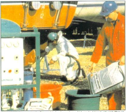
Goodchild Marine operates the Sponge-jet cleaning system, which can be taken to site and offers an environmentally-friendly alternative to conventional blast cleaning.
