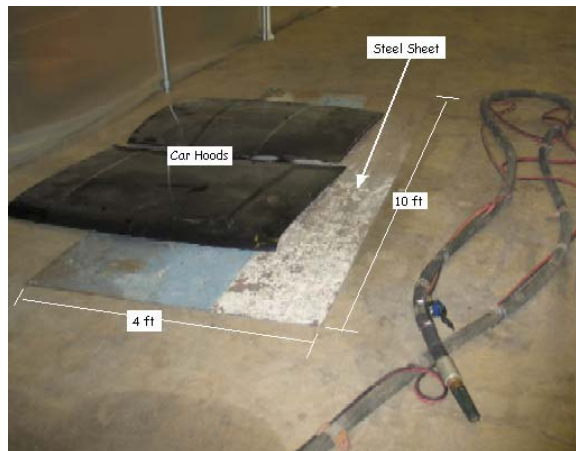
Photo 3. Blasting Area Inside Tunnel
