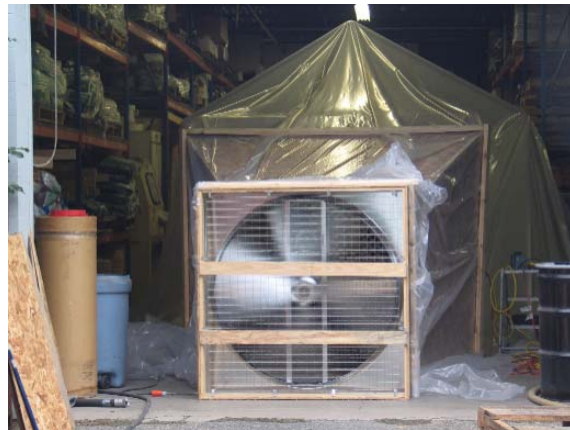
Photo 2. Exhaust Portion of Tunnel
