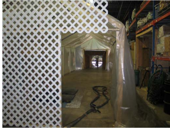
Photo 1. Looking Downstream From Tunnel Entrance (Latticework removed for access)
