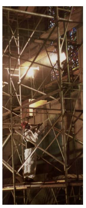
Church officials searched for a quick, dry, sensitive process that would remove fire damage and aged contaminants from walls, ceilings and trim of the New York City landmark.
